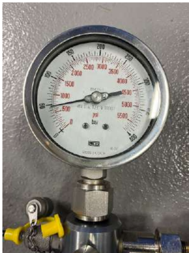
Figure 9: Test pressure reading
